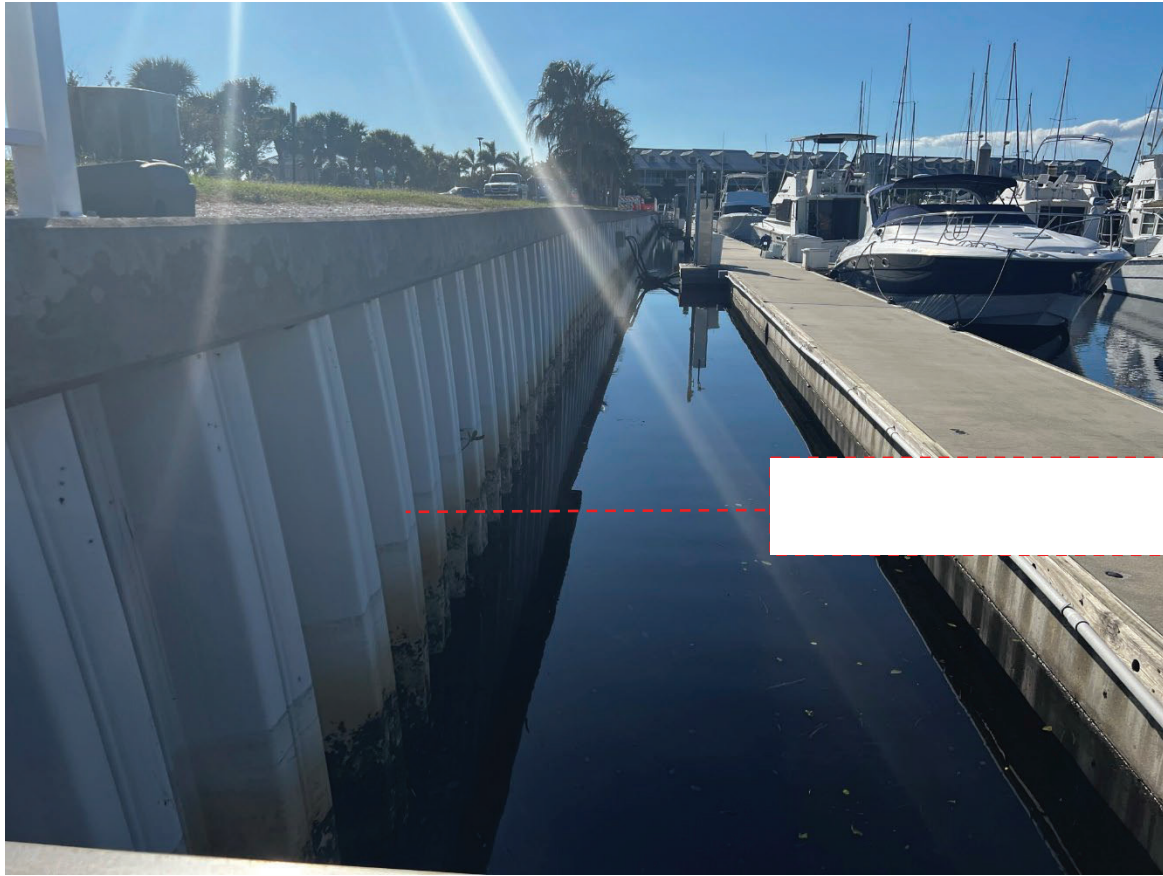
Photo #10 – Top View of Southwest End of Seawall Movement.
