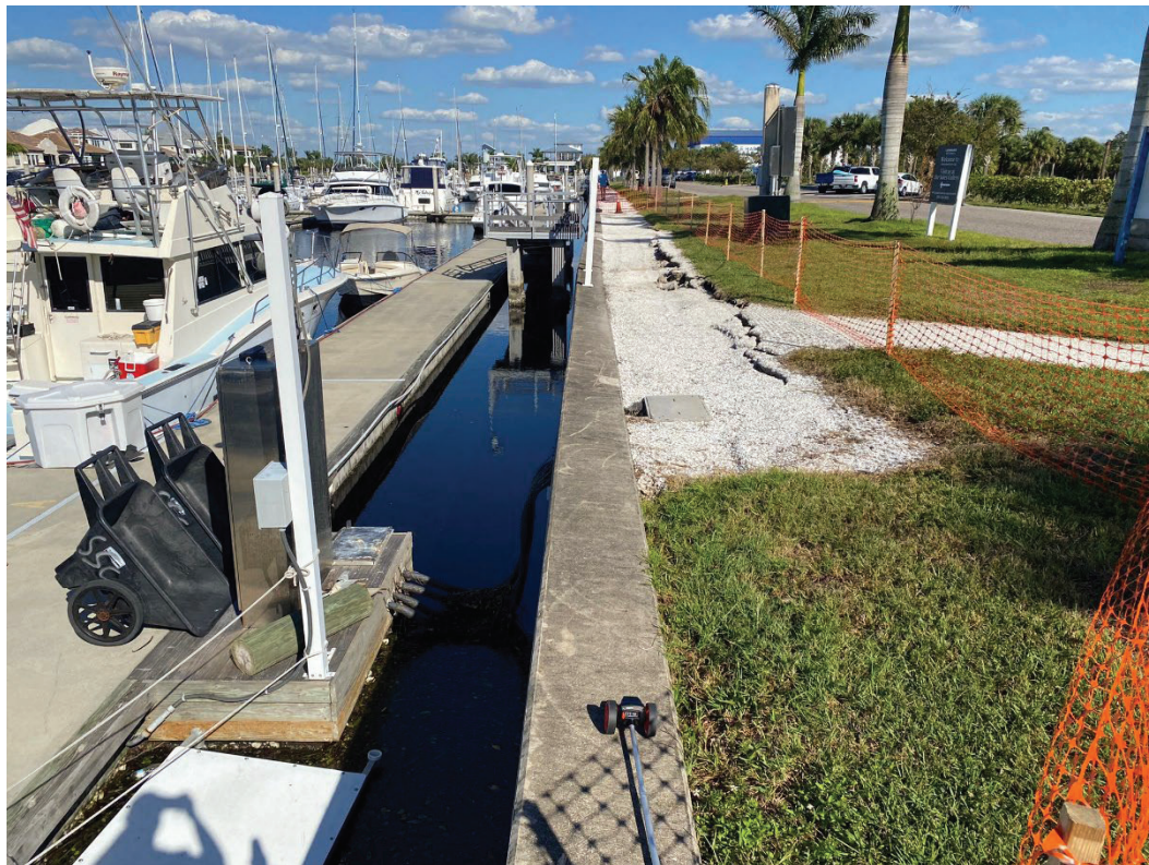
Photo #10 – Top View of Southwest End of Seawall Movement.
